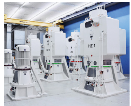
Walter Aeschbach is the head of the maintenance department at the Zurich Municipal Water Utility. At the Hardhof waterworks, he proudly presents the Sulzer pumps that transport the groundwater.
