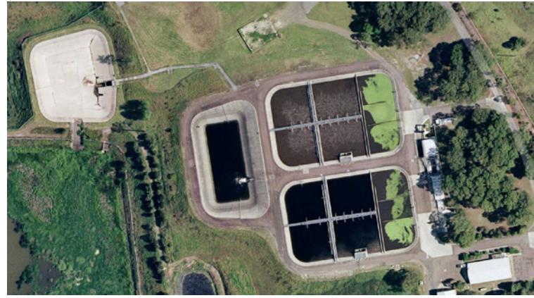
The Shortland wastewater treatment plant
